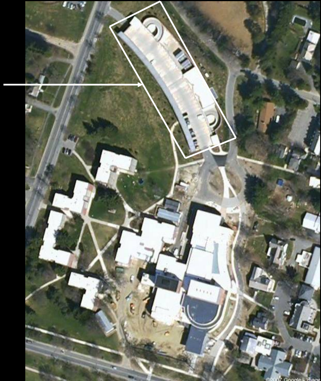
Aerial During Construction
